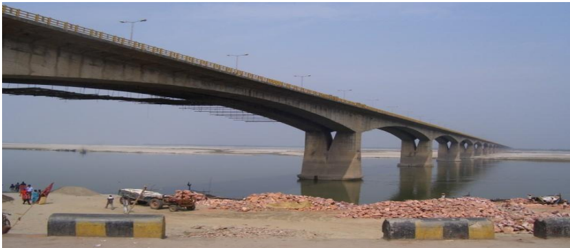
Ganga Bridge at Patna
