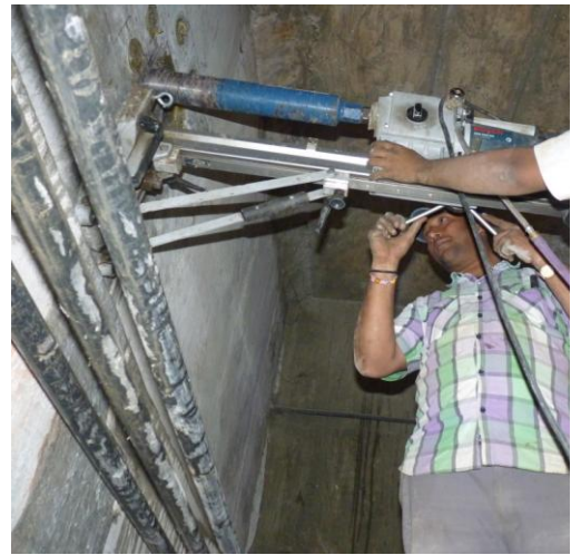
Core cutting on Girder
