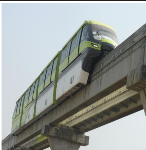
Field testing of Mono rail Project
